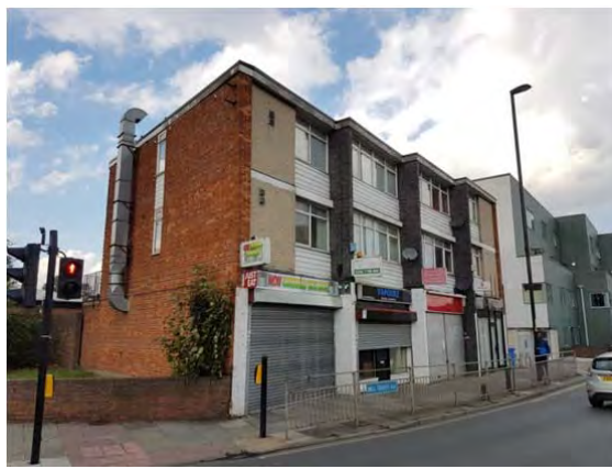
South and East (front) elevations
