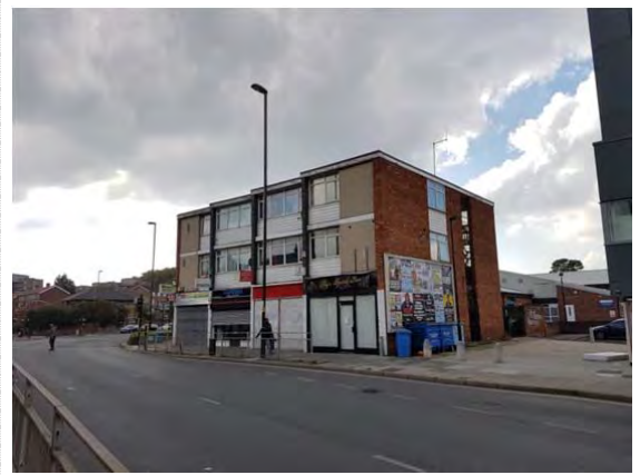
East (front) and North elevations
